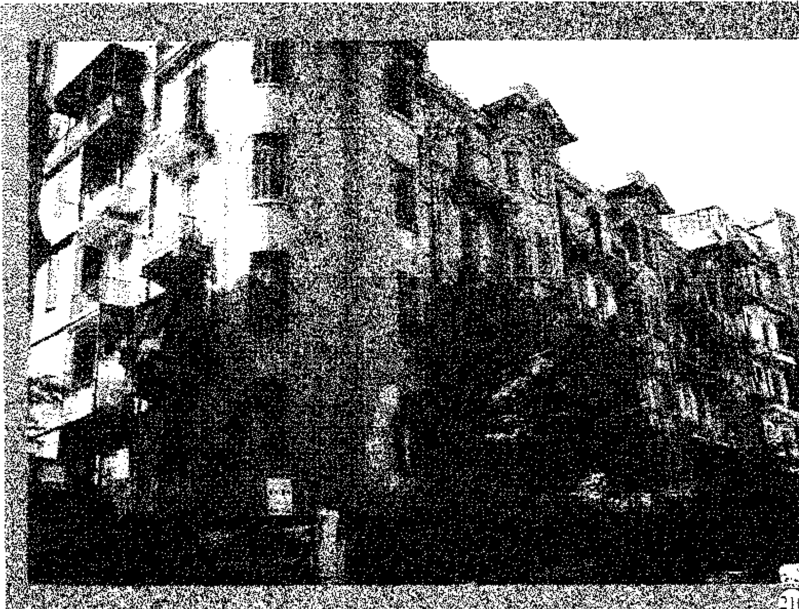
14 & 16 El-Kanisa El-Morqusia St. Built : about 1930 Area : 365 m 2 (both buildings) No. of storeys : 5 Style : Art Deco & Expressionism Influence
